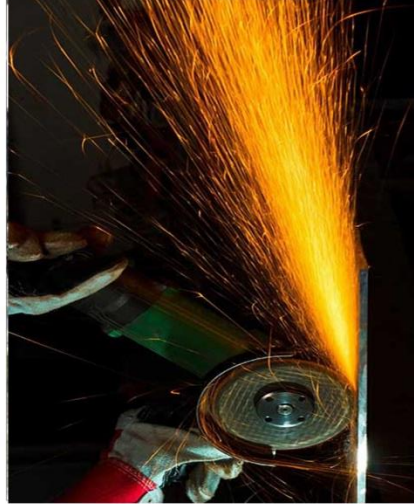
Welding work in Jizan IRTP (TR-10) Naseer Saeed Al-Hajri & Partners Company-2017 & 2018
