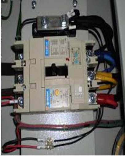
Cable Termination work in Jizan, JSRU (PKG-1&2) Consolidated Contractors Company (CCC) 2017 & 2018
