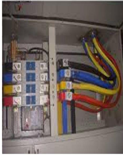
Cable Termination work at Jizan JRTP (TR-10) Nasser Saeed Al-Hajri Corp. 2017 & 2018
