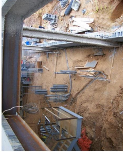
Conduit work at Ummal Sub-Station Dammam Saudi Electricity-2017
