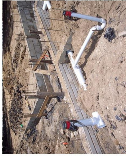
Plumbing work in Dammam Arkan Plastic Factory Kanooz Project-2017
