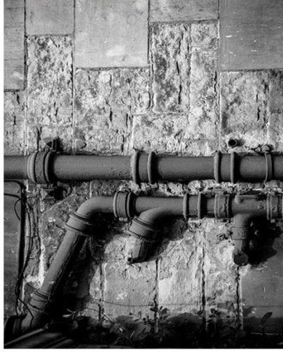
Plumbing work at Ummal Sub-Station Dammam Saudi Electricity-2017
