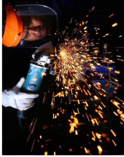
Welding & Grinding work in Jizan JSRU/SARU (PAK-1&2) Consolidated Contractors Company (CCC)-2017-2018
