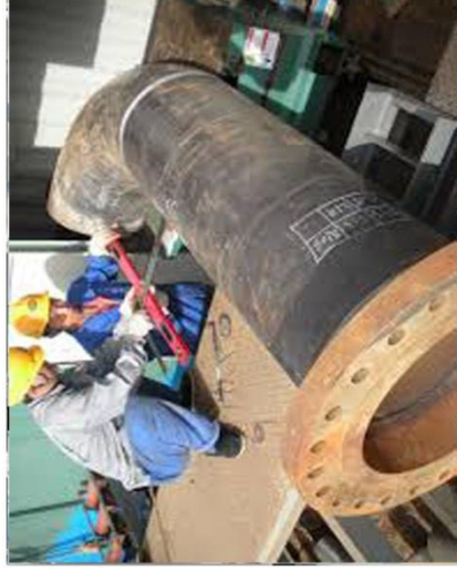
Pipe Fitter work in Al-Hasa Arabian Metal Factory Co. Ltd. (AMFCL)-2015
