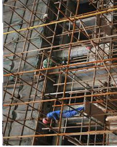
Scaffolding work in Jizan JRTP (TR-10) Naseer Saeed Al-Hajji & Partners Company-2018
